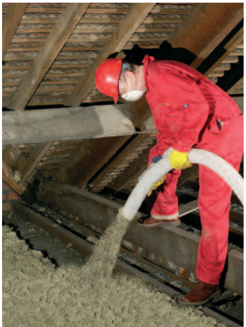
Installation of Rockwool Blown Loft Insulation
