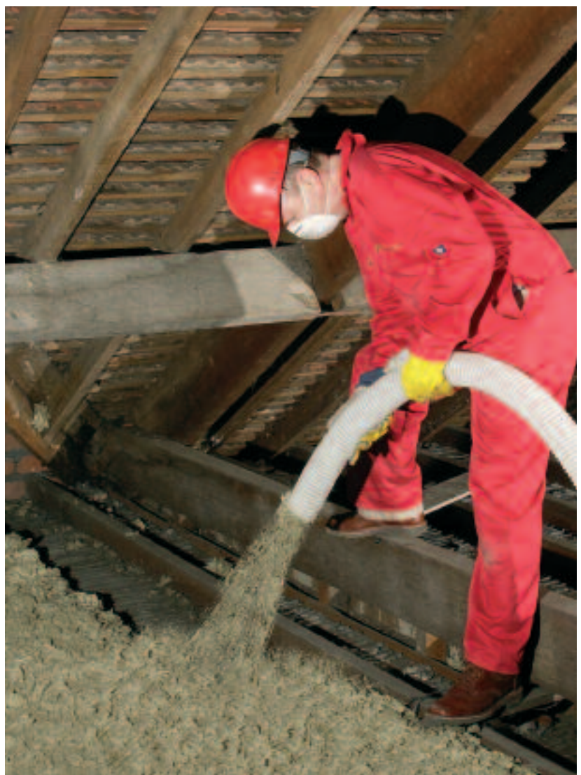
Installation of Rockwool Blown Loft Insulation
